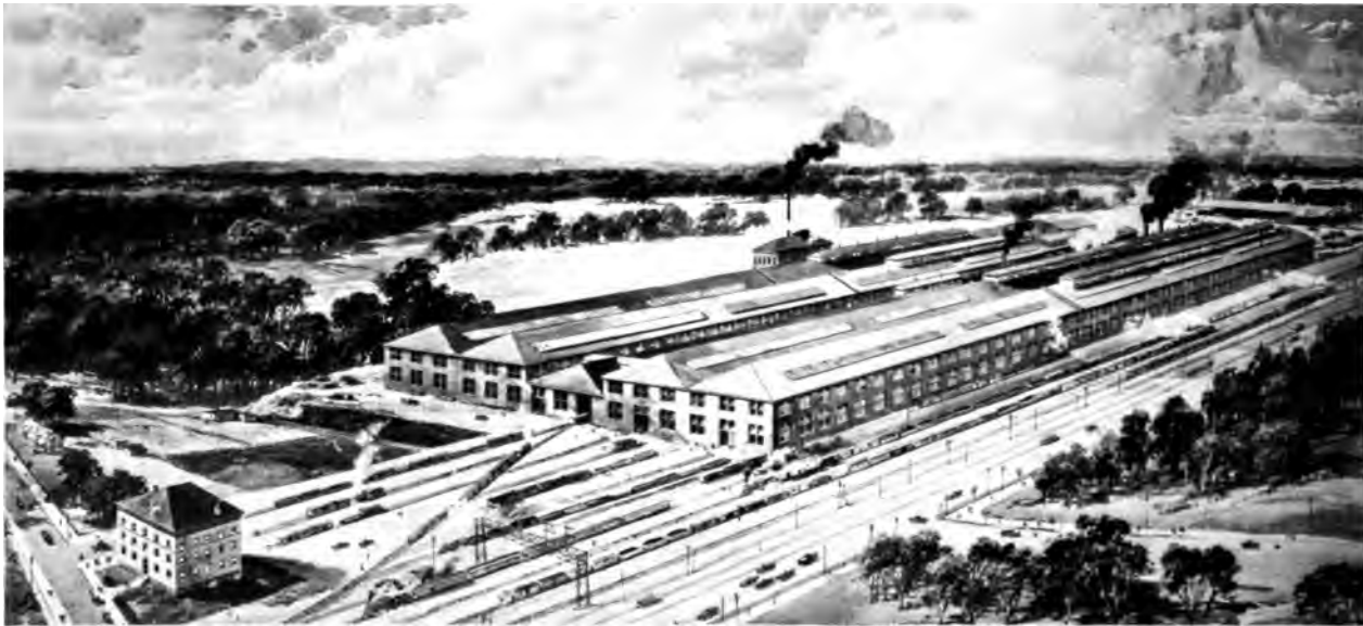
THE UNION SWITCH & SIGNAL COMPANY.
